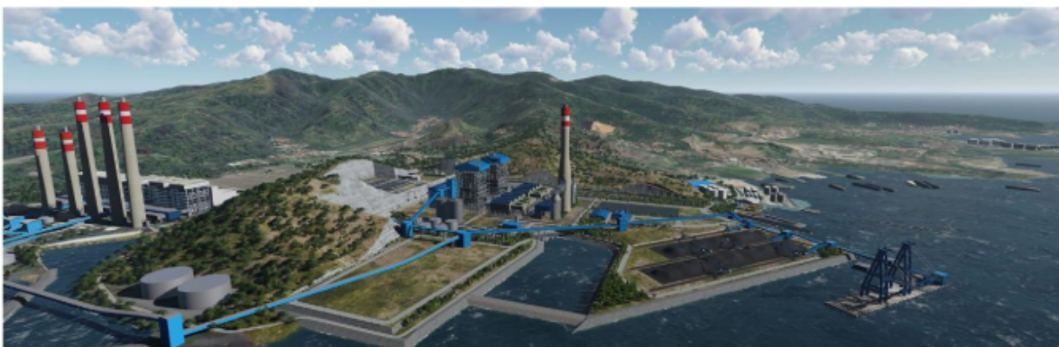
Figure 6. Suralaya Power Plant
